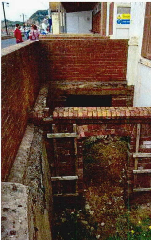
Levels at front of building
