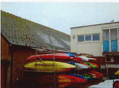
Boat store adjacent to rear of building
